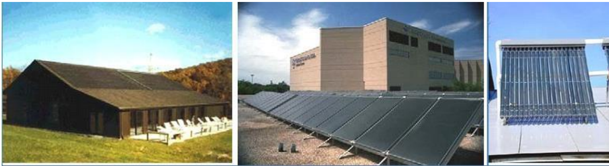
Fig. 6. From left to right, examples of unglazed, glazed, and evacuated tube solar hot water systems
