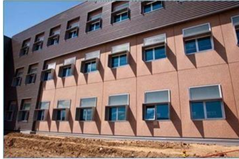
Fig. 8. The National Renewable Energy Laboratory Research Support Facility has a solar ventilation preheating system installed by the United States Department of Energy.
