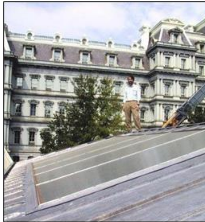
Fig. 10. The White House in Washington, DC has a solar water heating array built into its historically accurate, tene-coated copper, standing-seam roof.
